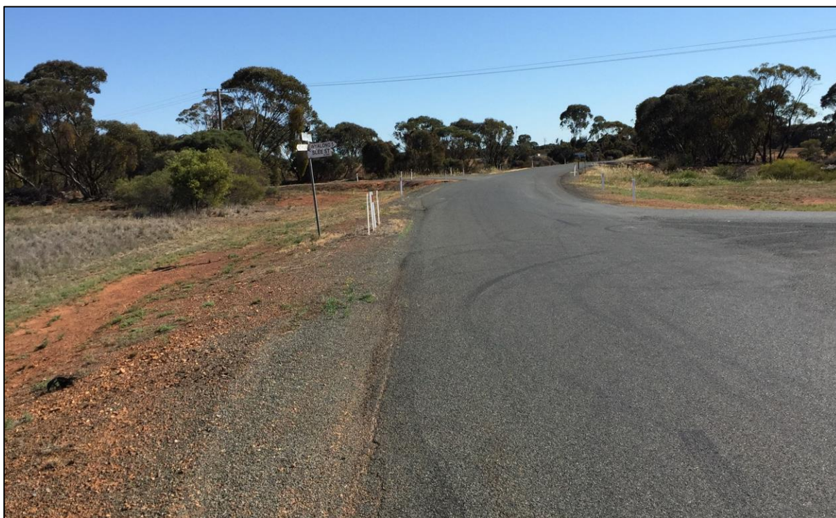
Figure 8: Clear Ridge Road at Slee Street
