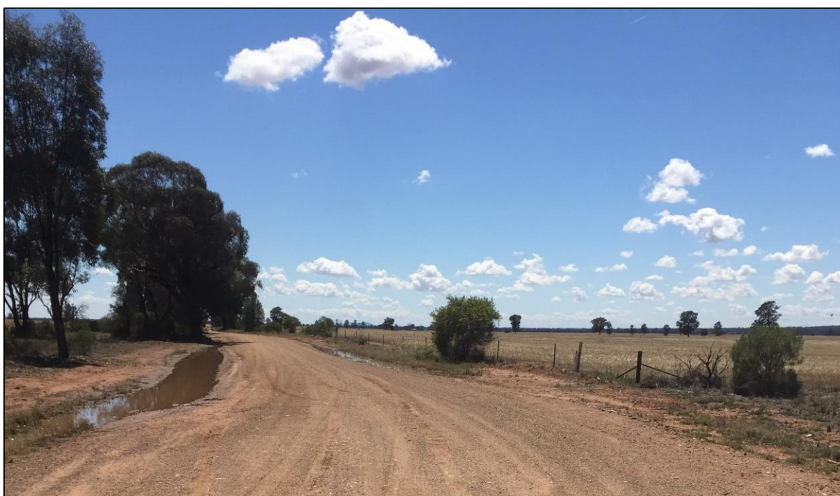
Figure 11: Blands Lane East of Clear Ridge Road
