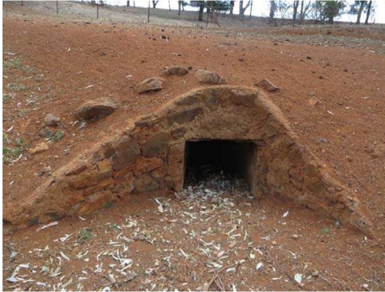
Figure 4-7 Man-made Culvert within the development site.
